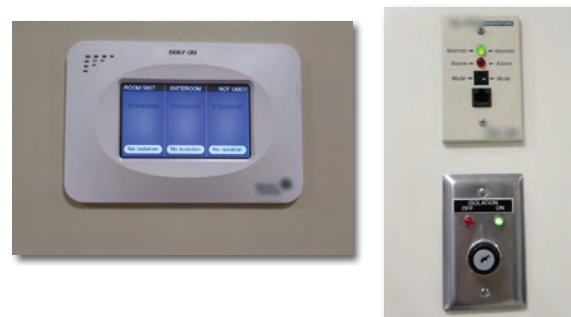
(left): A touch screen AIIR negative pressure monitor with visual and audible alarms that activate if the room air pressure becomes positive; (right): Another type of AIIR negative pressure monitor with visual and audible alarms
